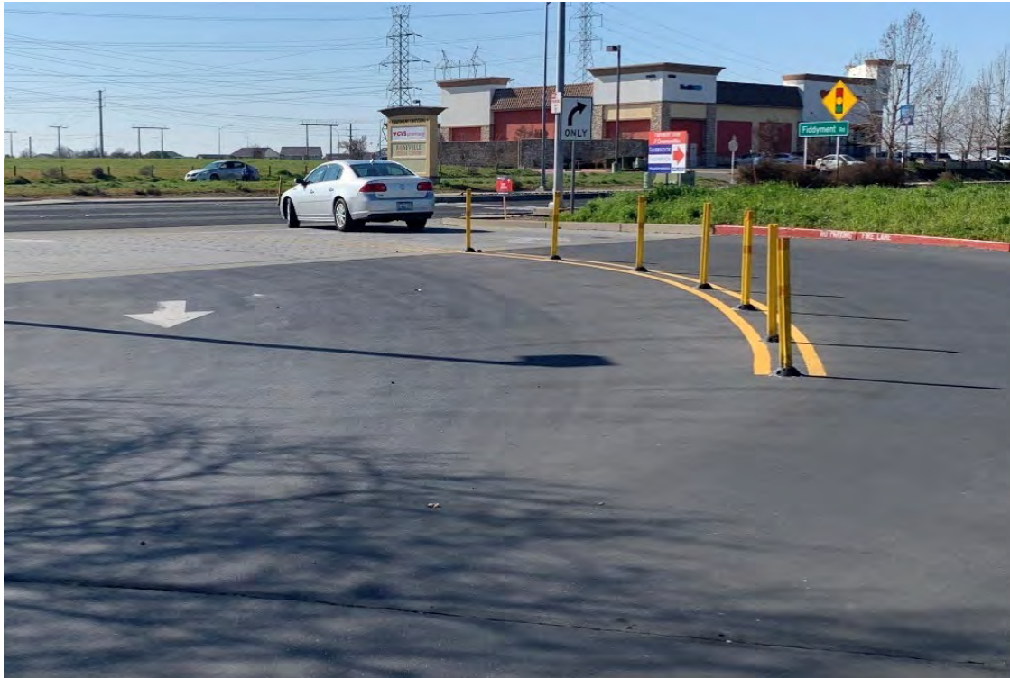
Photo of Driveway 4 exit onto Pleasant Grove Boulevard. Note signage prohibiting outbound left-turns.
